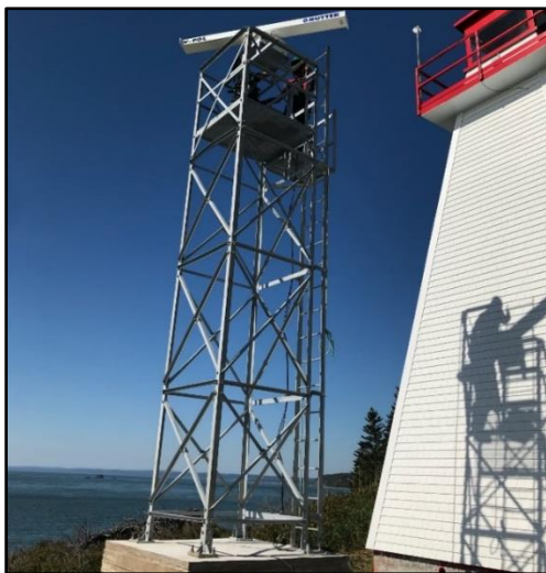
Figure 5: One of two high-resolution radars constructed near the FORCE site to be used for the Risk Assessment Program.
